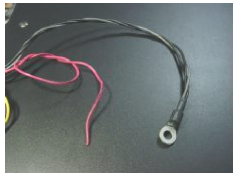
red wiring : +batt (back up power)
